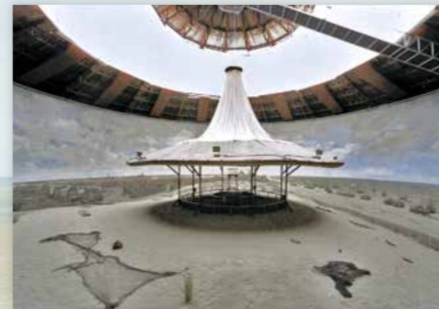
Principle of the Panorama: daylight falls upon the circular painting whereas the spectators stand under the cotton awning.
